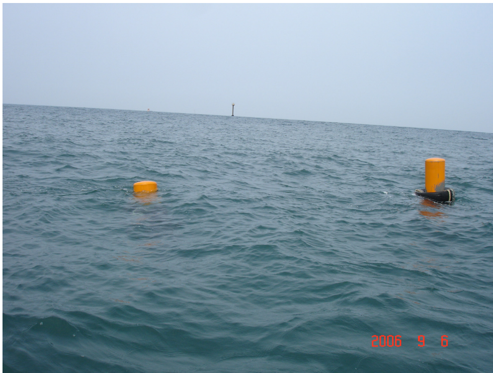
Photo B A semi-closed pipe after installation (半封閉圓管安裝完成後情形)
